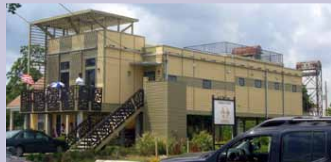
Rebuilding in the Lower 9th Ward Photos by Matthew Rufo
