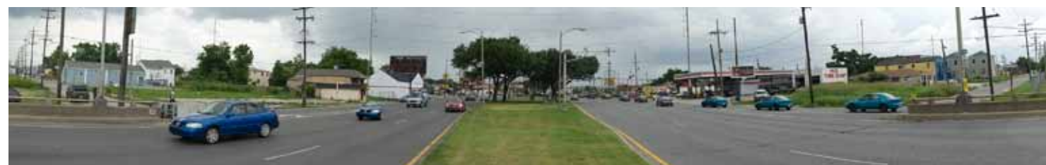
S. Claiborne Avenue can best be characterized as an auto-dominated, underutilized commercial corridor. Photo by Rami Diaz
